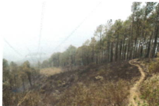
Forest Fire between tower span 41 to 42
