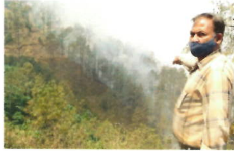
Forest Fire between tower span 5 to 6
