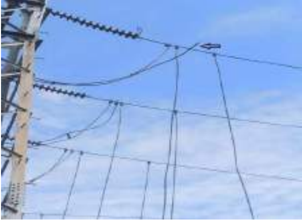
Damaged conductors at dead end and CVT jumper
