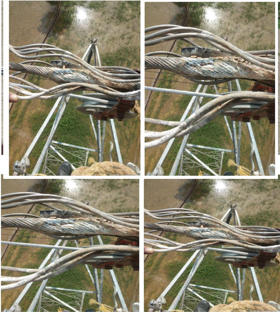
Fault on OPGW Cable in Agra- Ballabhgarh Link
